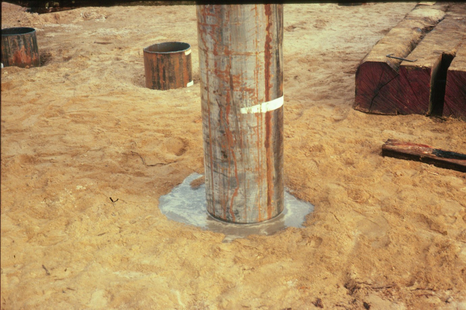
Driving closed-toe pipe piles into fine sand about 2.5 m above the groundwater table
