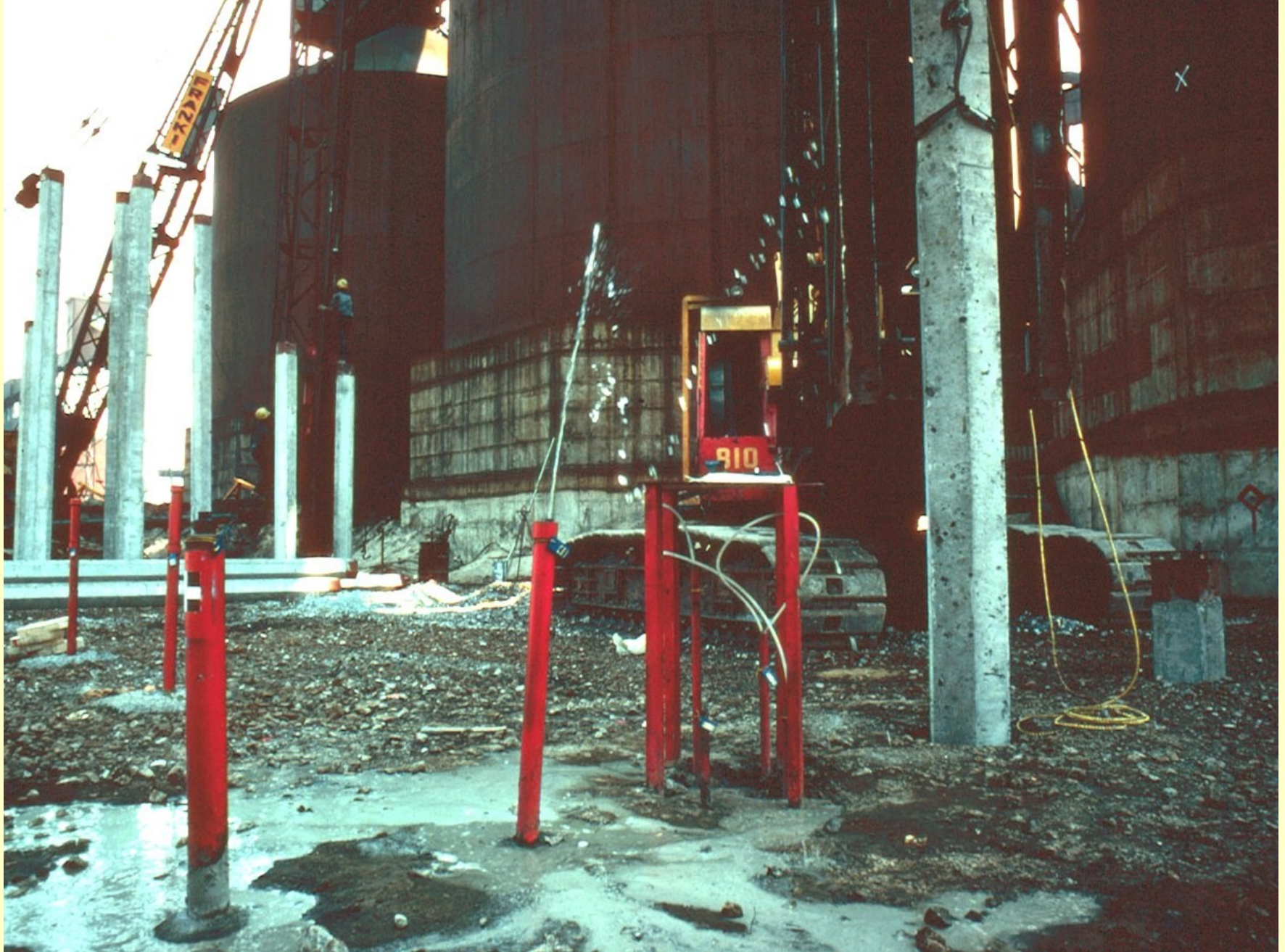
Driving 12-inch precast concrete pile into clay for Sidbec in 1974
