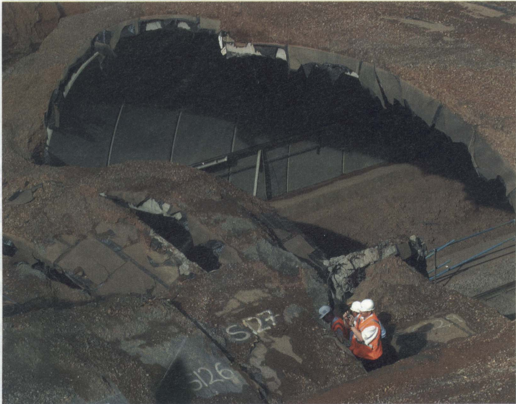
The collapse happened because not enough fill had been placed to the sides of the tunnel before material was placed on the crown.
