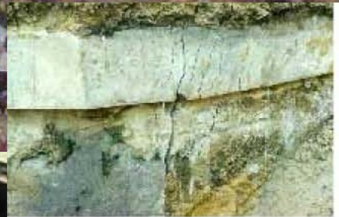
Cracks in capping beam
