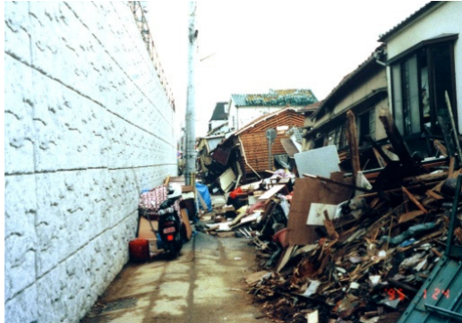
Figure 6 A GRS RW having FHR facing at Tanata, Kobe city, one week after the 1995 Kobe Earthquake (Tatsuoka et al., 1997a, 1998)
