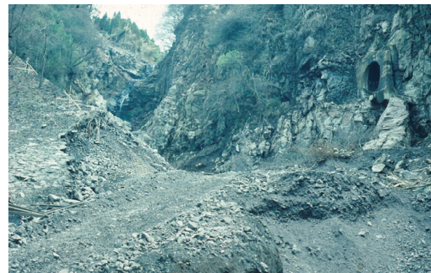
Figure 18 a) Locations of three major embankment failures by heavy rainfall in 1990 (site C in Fig. 5a), Hohi Line, JR Kyushu; and b) a view from the downstream at site 2 (Tatsuoka et al., 1997a)
