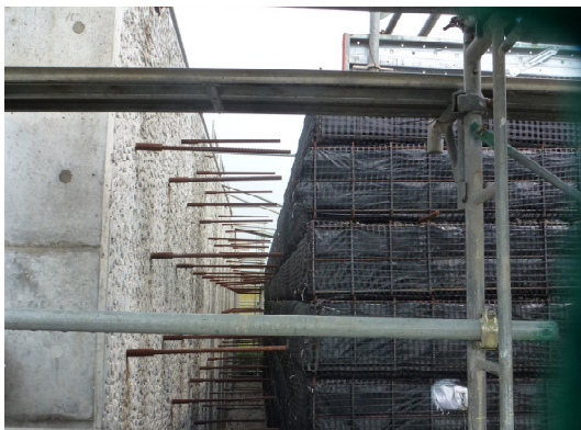
Figure 15 GRS culvert box culvert for Hokkaido Shinkansen: a) general structure; the numbers denote the construction sequence (site B2 in Figure 2b); and b) a space between the RC box structure and the approach block before step (3) (site B1) (Yonezawa et al., 2013)
