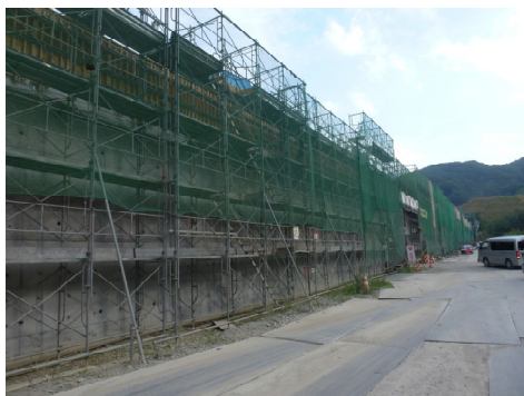
Figure 3 A view at stage 6 in Figure 1a of GRS RWs at both sides of a box culvert, site B2 in Figure 2b (Yonezawa et al., 2013)
