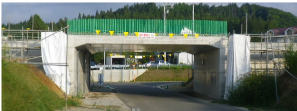
Figure 14 GRS integral bridge at Kikonai, Hokkaido Shinkansen (at site I in Figure 2b)
