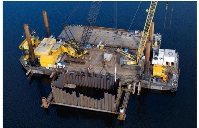
Figure 16 Water-filled caisson constructed of sheet-piles in foreground. In background, the barge is seen from which compaction was carried out, from Massarsch et al. (2017b)
