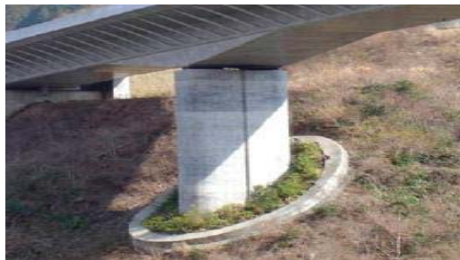
Figure 5 Photo of bamboo-cutting method of shaft foundation
