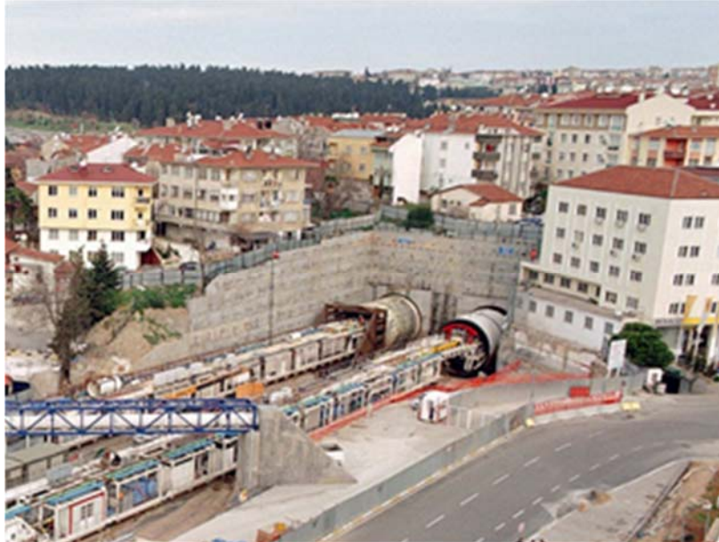
Fig. 5-2 Excavation in an urban area
