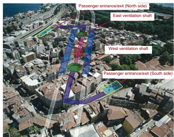
Fig. 4-1 Land use directly above Sirkeci Station
