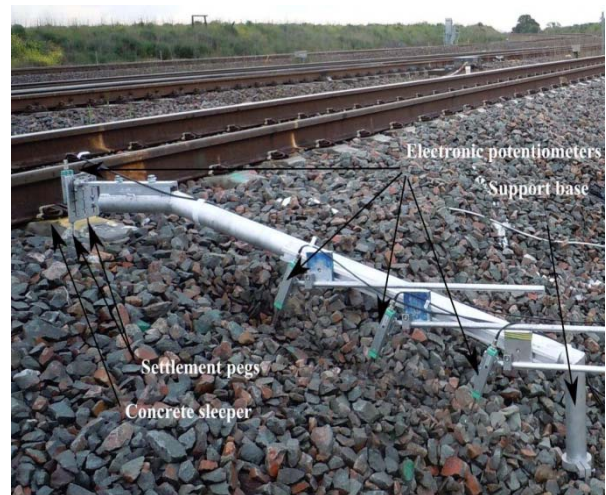
Fig. 2 Track displacement Monitoring (Indraratna et al , 2014)
