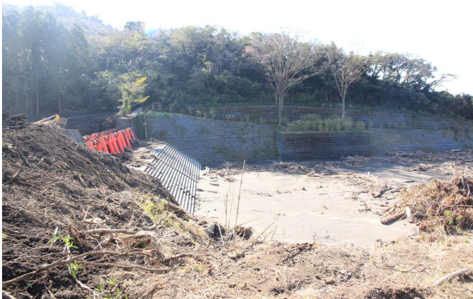
Fig. 7 Catchment dam for debris flow
