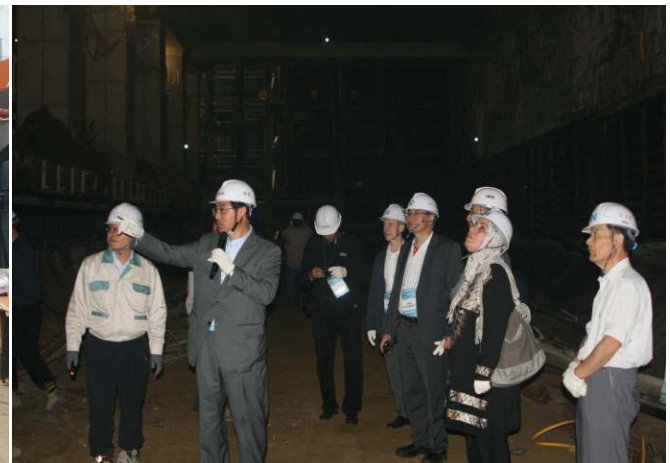
Photo 25. Incheon Metro Construction Site by Korean Tunneling Technology, TRcM
