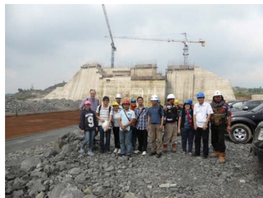
Picture 38 Participants on the highest fill placement (the spill way and core of the dam in the background)
