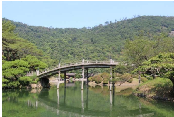
Photo 3 Scooping-the-Moon House seen under Crescent Bridge (偃月橋)
