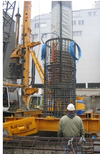
Installation of Energy Pile
