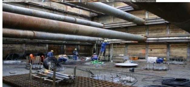
Installation of heat exchanger pipes and connection through raft
