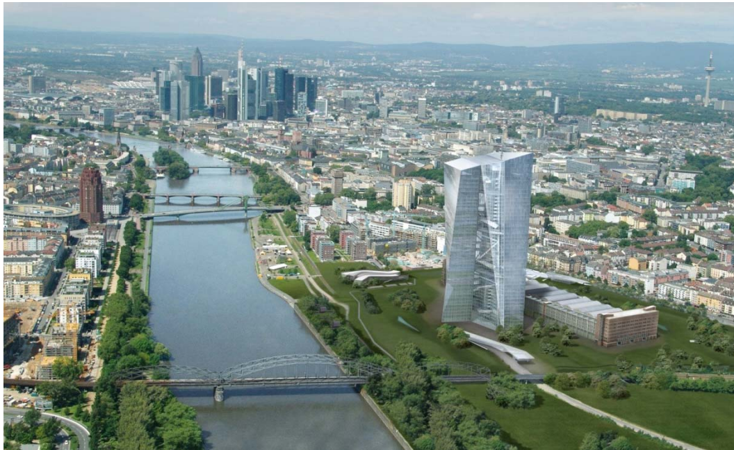
Skyline of Frankfurt am Main, Germany with several tall buildings having deep foundations
