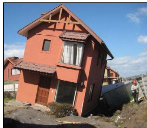
Fig. 12.- House in Talcahuano
