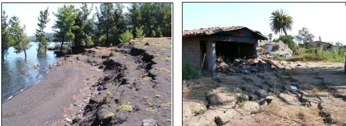
Fig. 9.- Lateral spreading observed in Calafquén Lake and Nancagua
