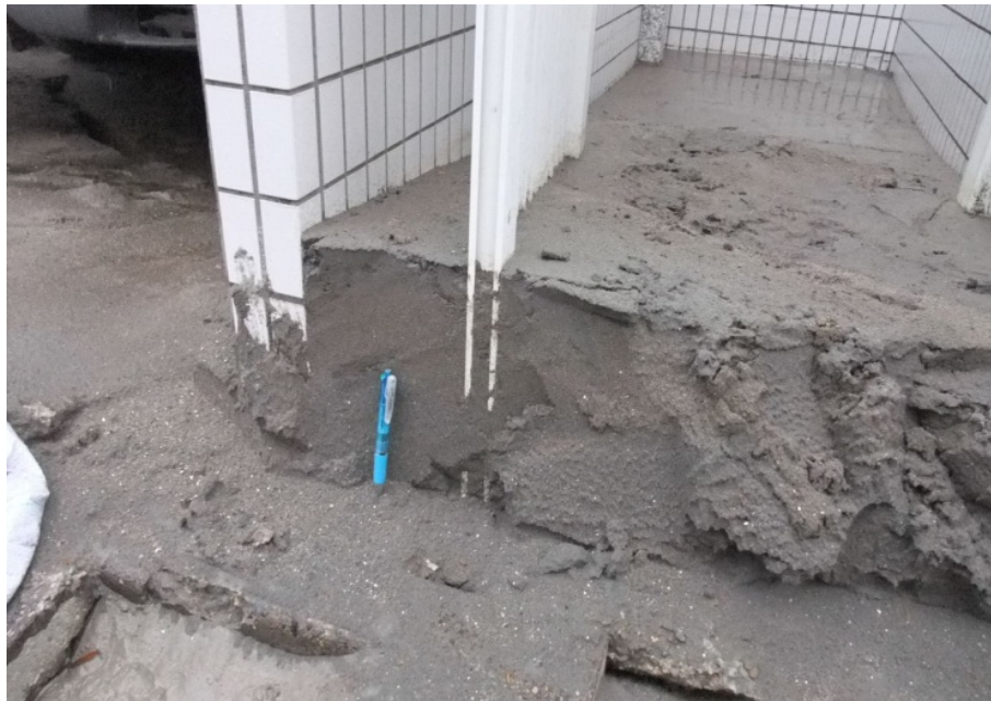
Photo 7 Thick deposit of ejected sand observed in Urayasu City
