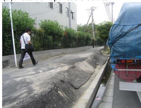
Photo 5. Distortion of sidewalk probably caused by subsidence of building behind
