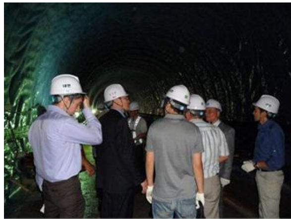
Incheon metro construction site
