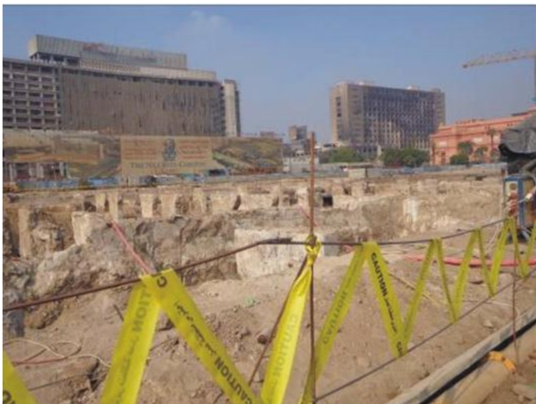
Ongoing Underground Multi-Story Garage at Tahrir Square
