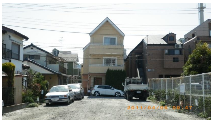
Photo 3. Tilting of house caused by liquefaction in a manmade island in the Tokyo Bay area
