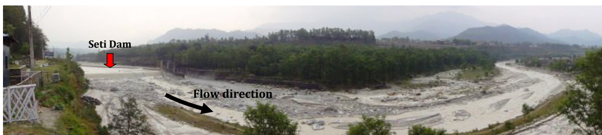
Fig. 6: Seti Dam area, about 4 km upstream from Pokhara city center (most live videos and photos of the flood freely available in the net were taken at this point). The dam structure has sustained the damage, mainly because at this point the debris was composed of less destructive material such as tree logs and finer particles.
