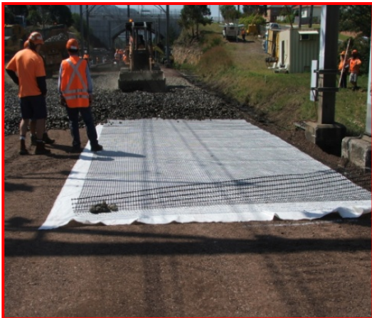
Rail Track improvement using Geosynthetics.
