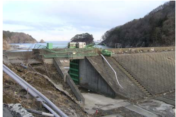
Fig. 22 High sea wall against tsunami attack (Karani-Hongo).
