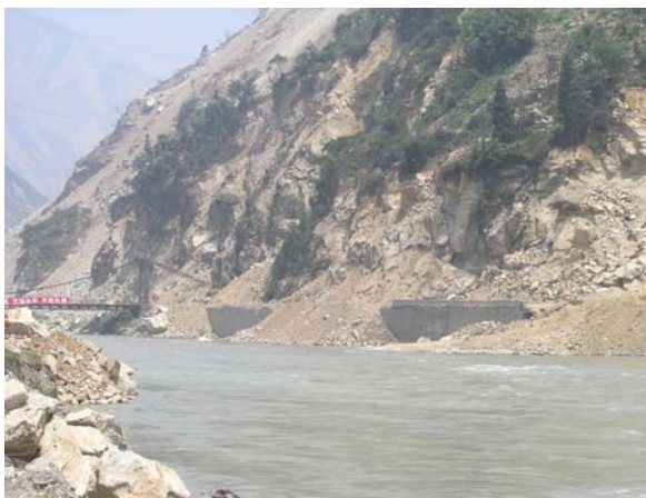
Fig. 5 Slope failure that occurred during the 2008 Wenchuan earthquake.
