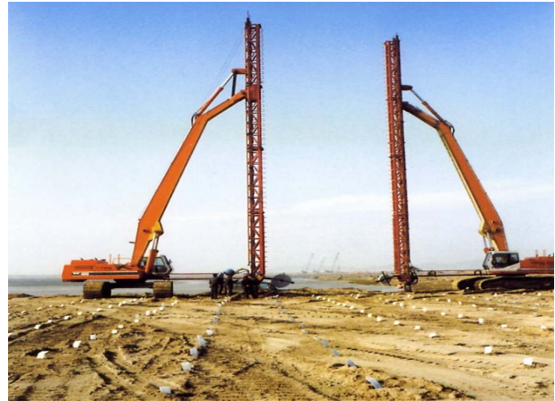
Port Reclamation using Vertical Drains
