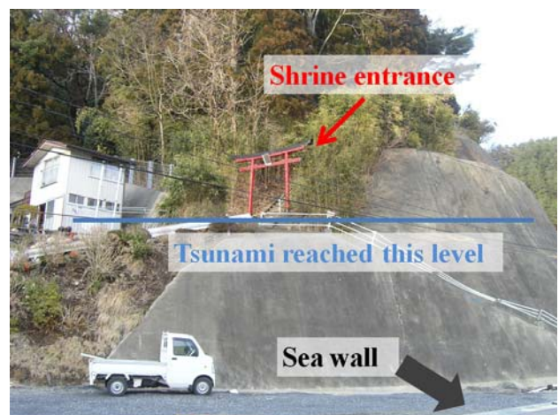
Fig. 24 Tsunami water level well above the sea wall and close to the entrance gate of a local shrine.
