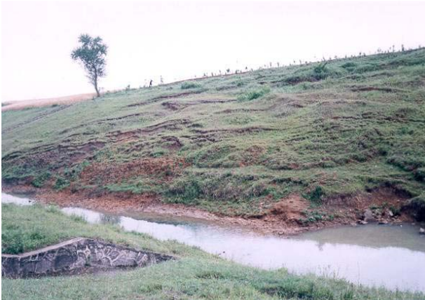
Figure 4 Typical shallow retrogressive failures at Dagangpo
