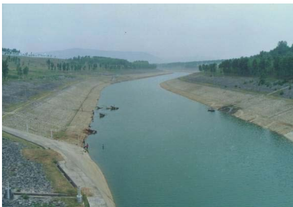
Figure 2 Intake canal of the Middle Route in Nanyang, Henan
