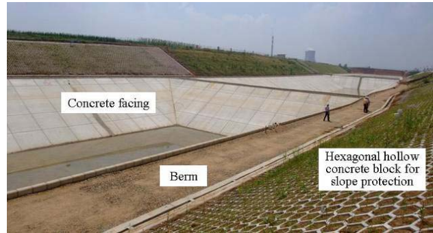
Figure 14 Part of Nanyang test section in expansive soil (Cheng et al. 2011)
