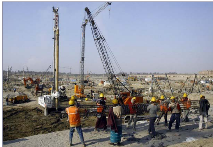
Figure 10 Piling in Progress at Site
