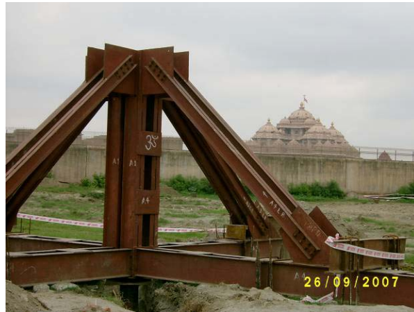
Figure 9 Pile Load Test Setup (See the Akshardham Temple in the background)
