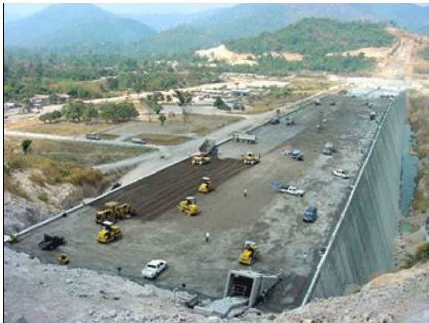
Fig. 10 Thadan dam - during construction
