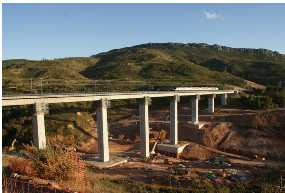
The viaduct of Pont de Candi being repaired
