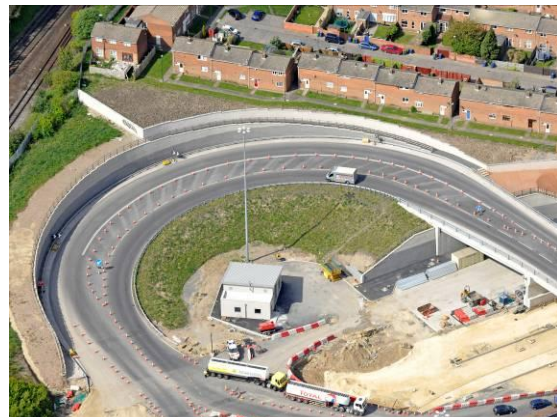
TensarTech TW1 Earth Retaining System uses site-won fill for walls up to 8m high and 200m long, UK
