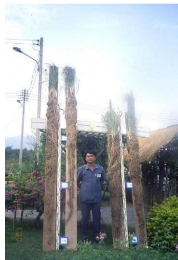
Fig. 12 Challenging situations for slope engineering in Thailand, Construction of reinforced soil slope, vetiver grass utilization and soil blanket in slope protection
