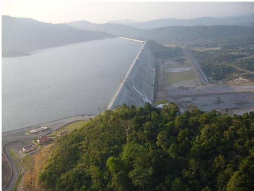
Fig. 11 Thadan dam - after completion
