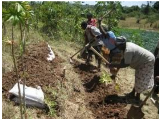
Figure 18 A terrace reinforced with "Do-nou" for the tree nursery
