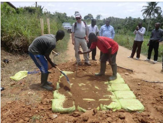
Figure 19 Prof. Kimura is supervising construction in Ghana
