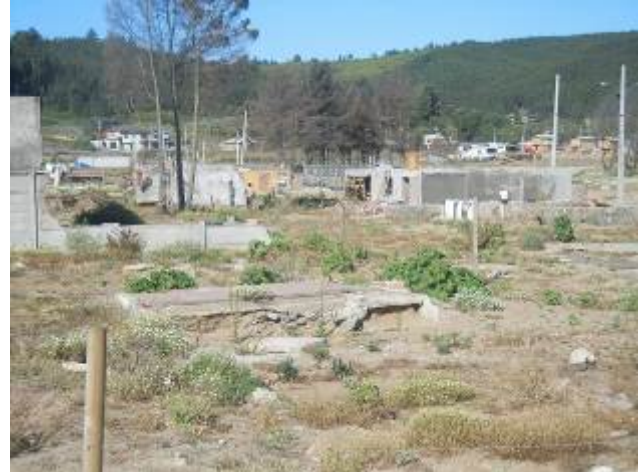
Site of Tsunami damage in Dichato
