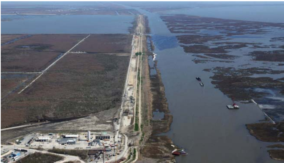
Figure 3 Overall view of the LPV-111 site
