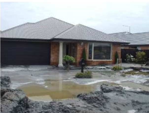
Photo 3 Repeated liquefaction near Bexley
