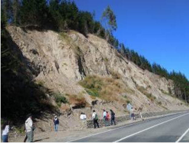
Failure of coastal slope near Concepcion
