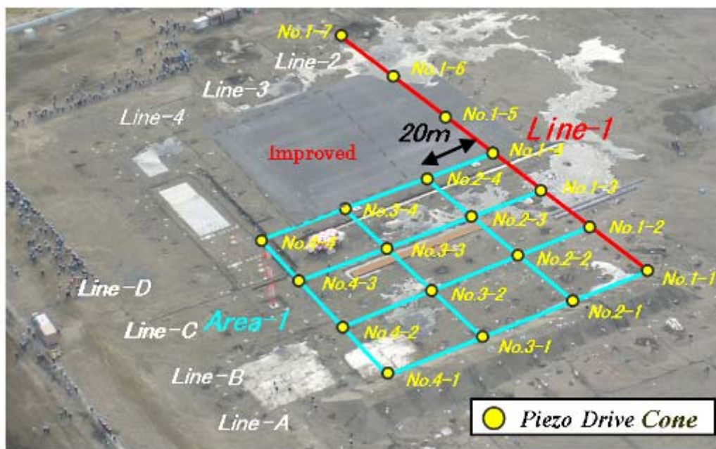
Fig. 15 Aerial view of site of preliminary field blasting.
