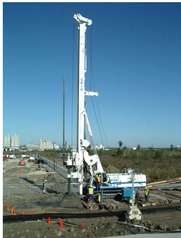
Figure 8. TREVIICOS Rig (Soilmec SR-70 - single shaft)
