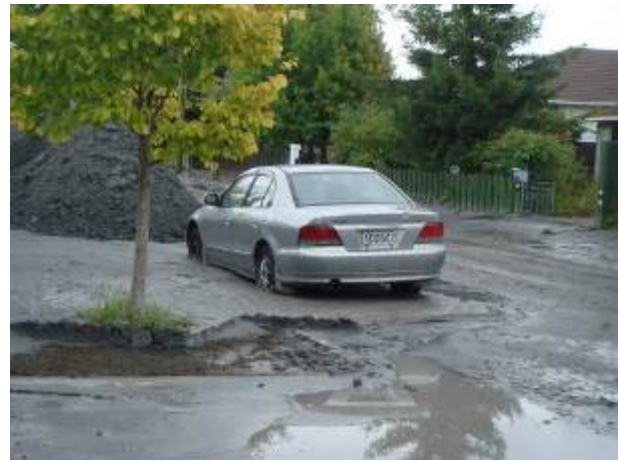
Photo 2 Liquefaction in residential area in Edgeware
