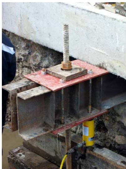
Figure 5. Underpinning piles support the whole structure
