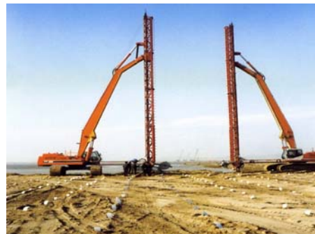
Port Reclamation using Vertical Drains
