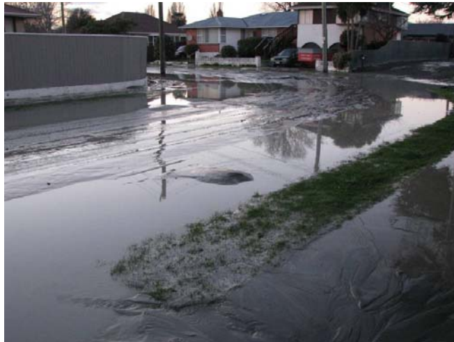
Photo 1: First light - liquefaction street scape in the neighbourhood
