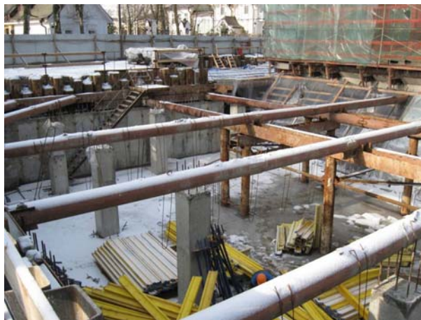
Figure 4. Underground construction outside the theatre footprint
