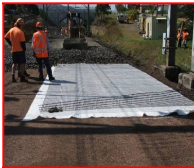
Rail Track improvement using Geosynthetics
