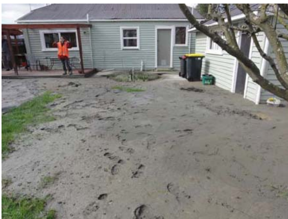
Figure 6. Evidence of extensive liquefaction (large sand boils) in residential areas of Avonside. Notice the chair embedded in 20 cm thick sand ejecta in the backyard of the property.
