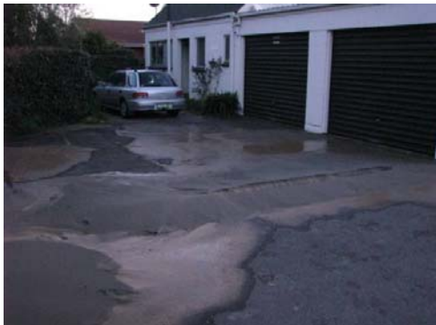
Photo 2: First light - a view of my driveway with liquefied soil and water
