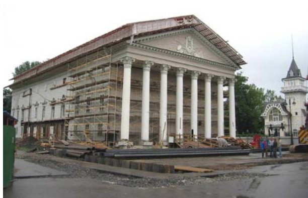
Figure 1. General view of the theatre during reconstruction
