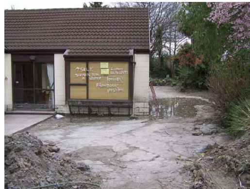
(a) ~40 cm thick layer of silt-sand-water mixture covering a residential property affected by very severe liquefaction; (b) same-angle view, but after the clean up of sand ejecta
