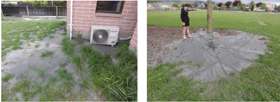
Figure 13. Sand ejecta at the perimeter of house foundations and in a park in Hoon Hay due to re-liquefaction during a M_w 5 aftershock; the aftershock occurred 45 days after the mainshock.
