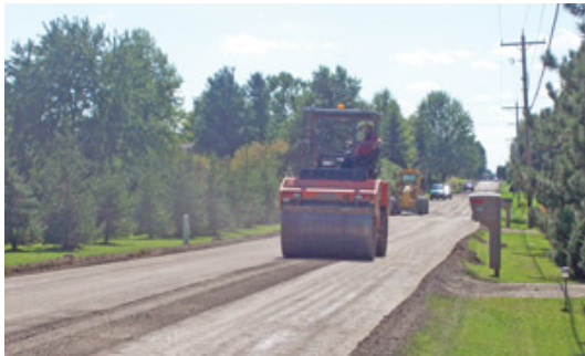
Figure 3. Compaction of FDR base
