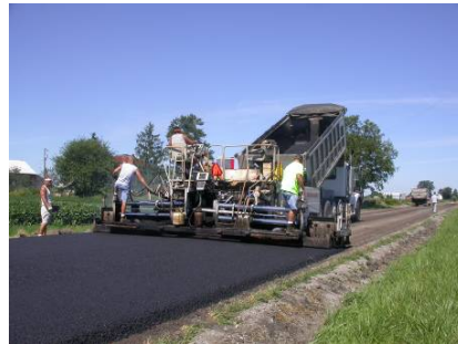
Figure 4. Resurfacing with hot mix asphalt
