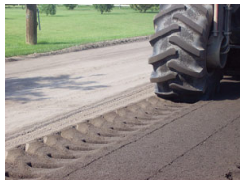
Figure 2. Blending fly ash with pulverized base
