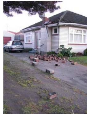
Photo 3: First light: typical chimney debris of a house in adjacent street
