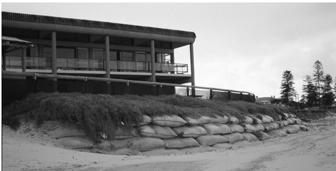
Figure 5. Revetment made with geotextile sand containers.
