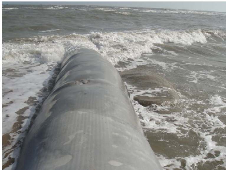
Figure 10. Groyne for prevention of coastal erosion
