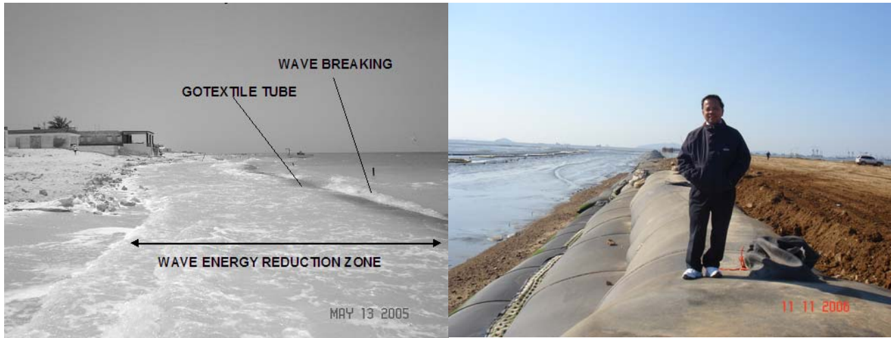
Figure 9. Geotextile tube inducing wave breaking for energy attenuation (Alvarez et al, 2005)
