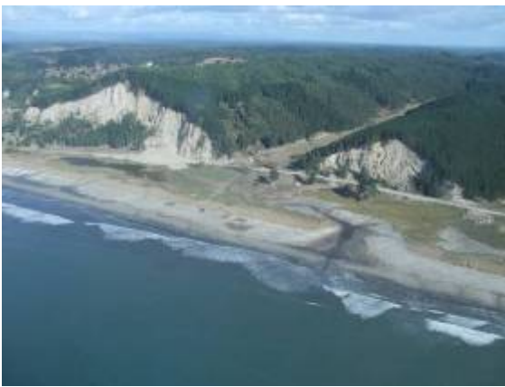
Photo 11 Slope failure at Las Peñas near Arauco
