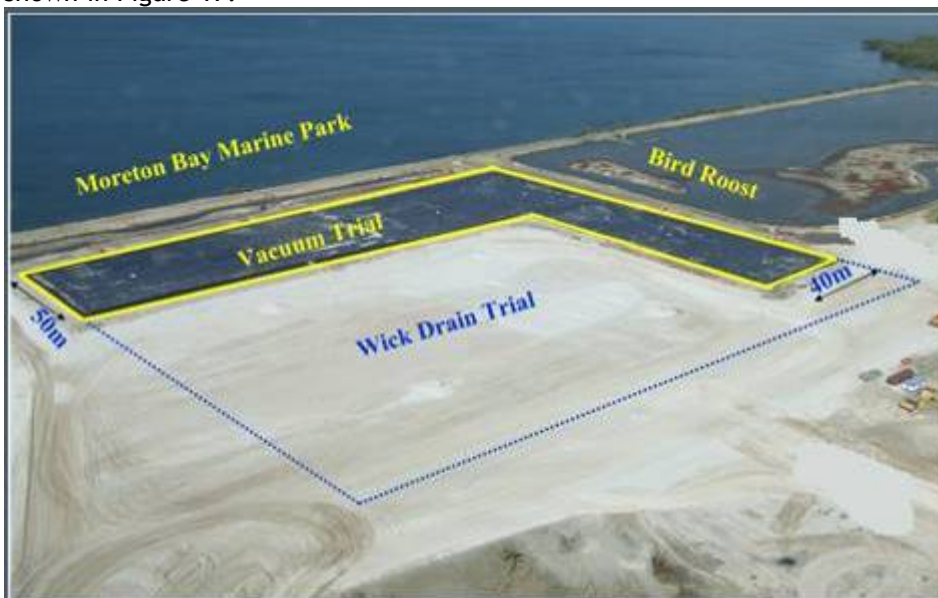
Figure 17 Menard Trial-Vacuum area with membrane placed and adjacent wick drain area
