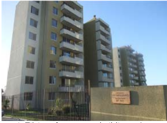
Photo 1 Tilting of apartment building at Los Presidentes
