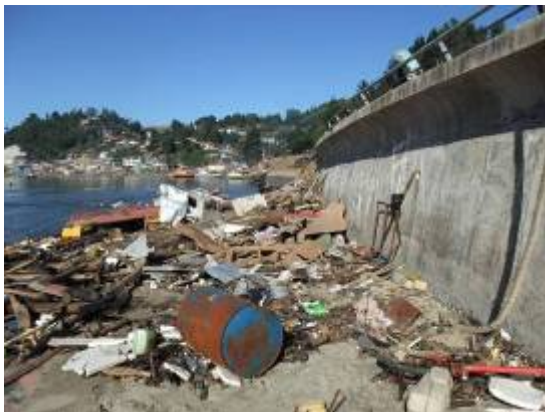
Photo 21 Successful performance of sea wall in Cape Blanca area.
