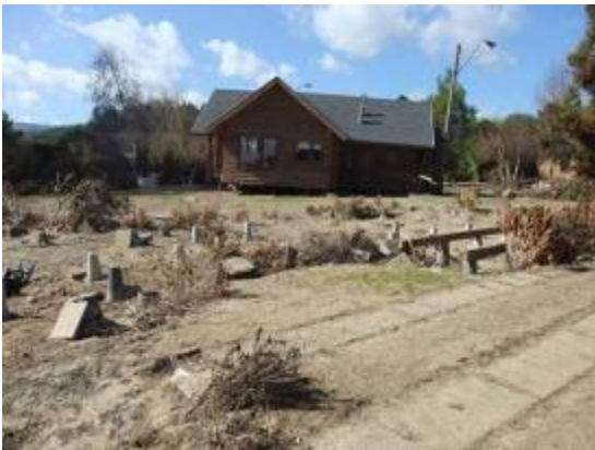
Photo 25 House that floated when tsunami came
