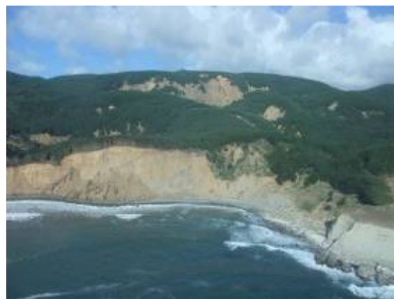
Photo 12 Slope failure at Lavapié
