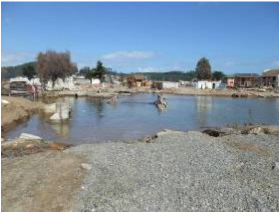
Photo 23 Tsunami-induced erosion in Dichato
