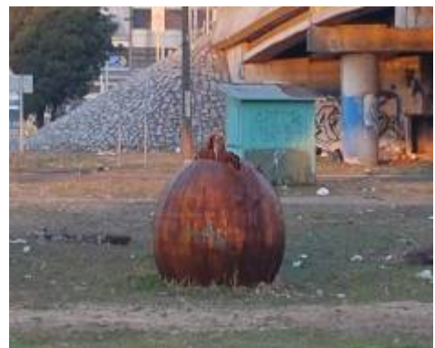
(Densification by dynamic compaction)
