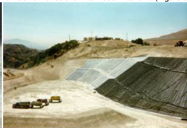
Figure 4. View of a liner system composed of geomembranes and GCLs in a waste containment project.
