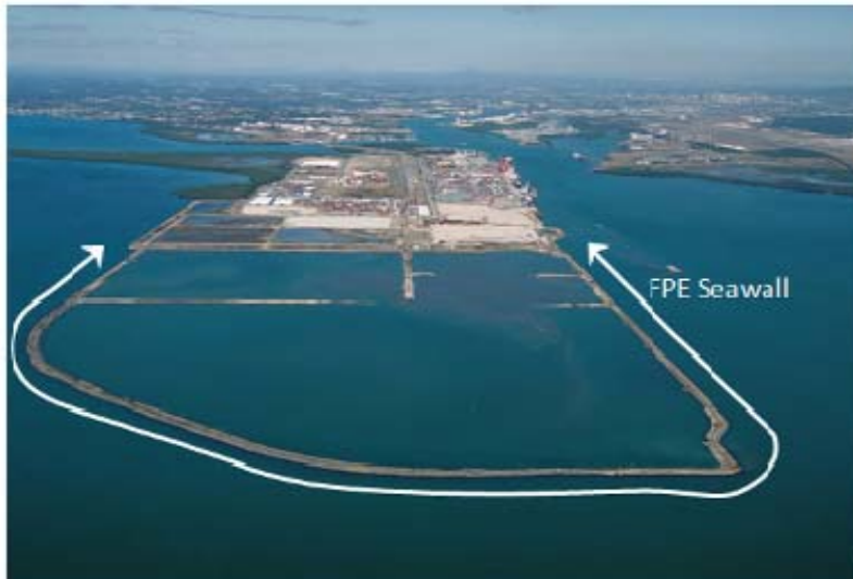
Figure 3: Future Port Expansion (FPE) Seawall - 2004
