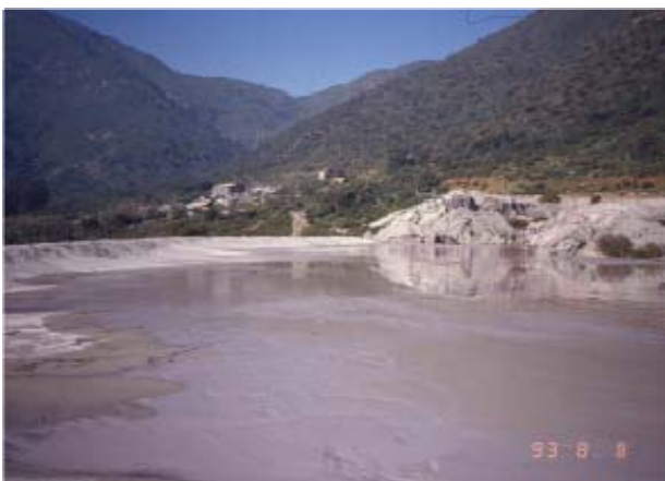
Photo 5 Reservoir of tailing dam at Veta del Agua in 1993.
