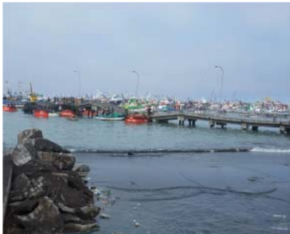
Photo 18 Damaged pier in Coronel
