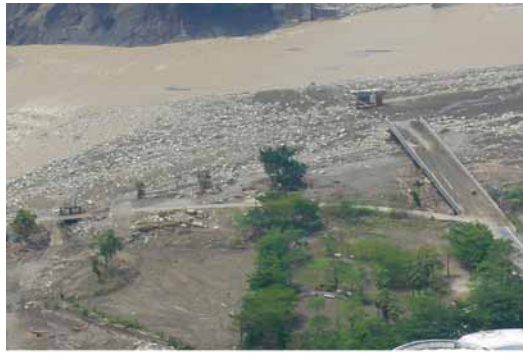
Figure 18. Destroyed bridge because of scouring
