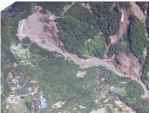
Figure 11. Aerial view of large slope failure
