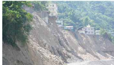
Figure 6. Erosion along river channel
