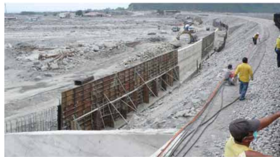
Figure 33. Reconstruction of railway bridge
