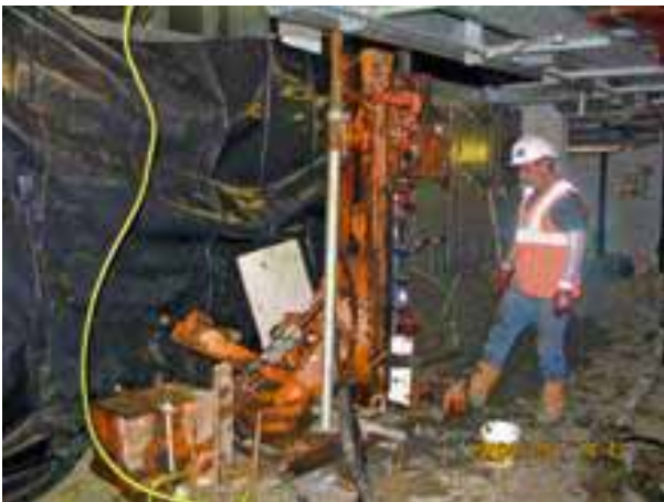
Figure 5: Probing and coring of existing UR piles
