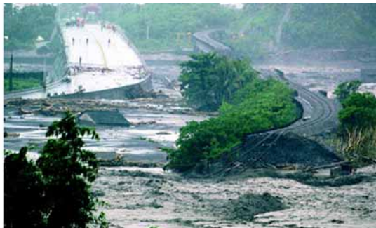
Figure 32. Bridges during flooding
