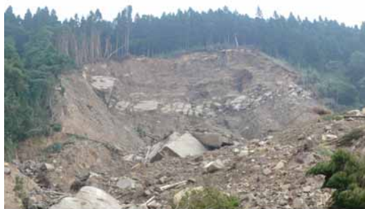
Figure 12. Deep-seated failure of slope
