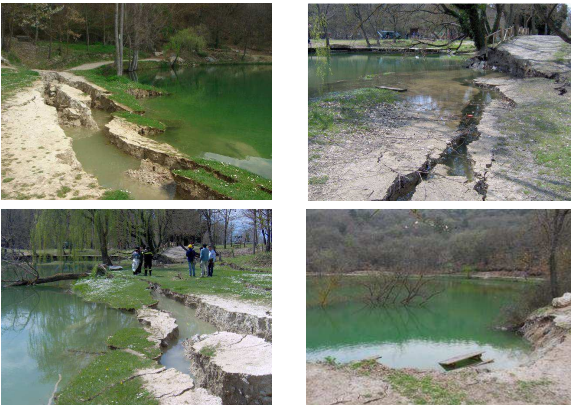
Figure 10. Lake Sinizzo near San Demetrio ne' Vestini. Ground cracks and large displacements along the eastern perimeter (above, left), northwestern perimeter (above, right) and western perimeter (below, left). Submerged trees along the western perimeter (below, right)
