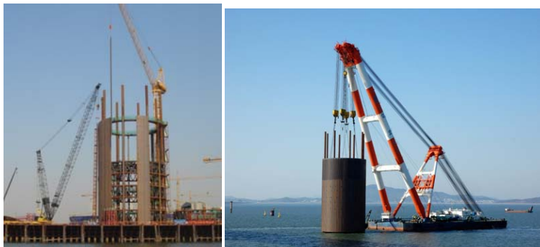
Figure 13. Fabrication and transportation of the dolphin cell
