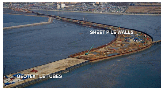
Figure 18. Geotubes and sheet pile walls
