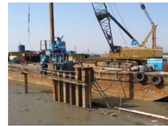
Figure 22. Push-in type sheet pile installation machines
