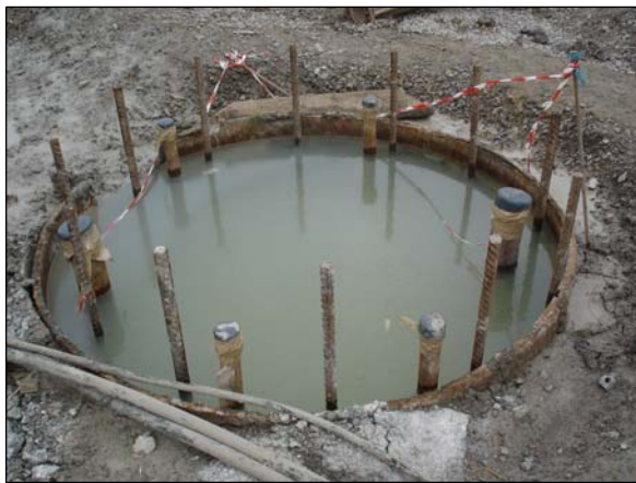
Figure 7. Pipes set up for shaft control
