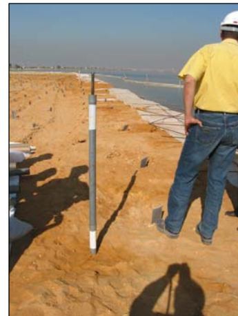
Figure 10. Installed geosynthetic drains and marks for settlement measurement
