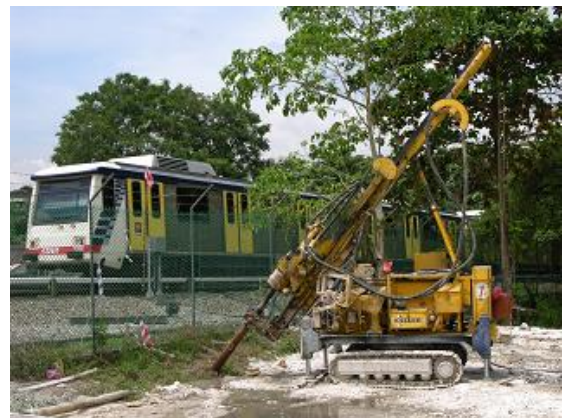
Fig. 5 Grouting treatment beneath the "live" rail track
