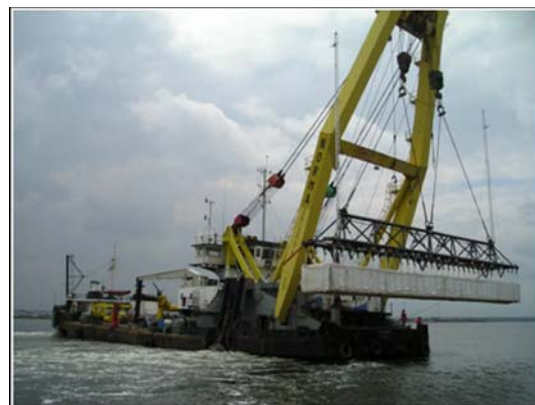
Figure 6b: Sand bags at installation on the underwater slope
