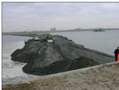
Figure 10: Situation dam at level TAW +4.5 m
