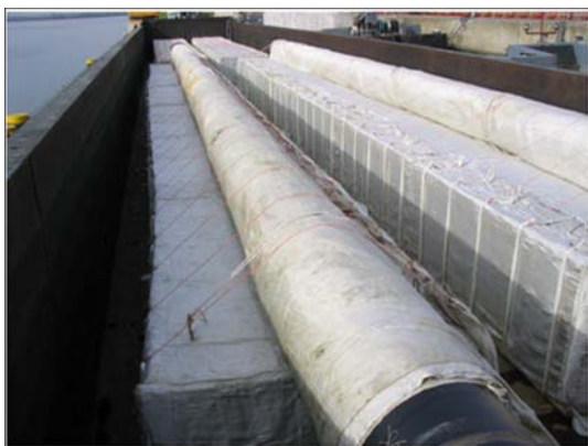
Figure 6a: Geosynthetics sand bags before installation
