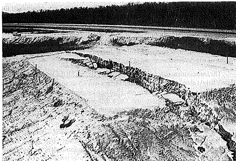
Fig. 5 General view of the embankment just after failure
